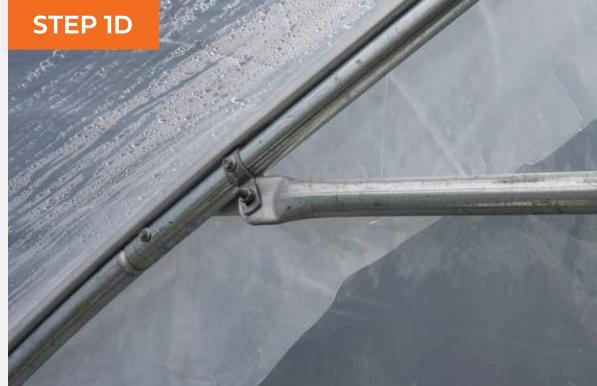
Attach the **Brace Bands (A1)** to the ends of the **Cross-Bracing Pole (A2)**.
